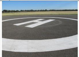
Marked by a large white H and circle and defines the helicopter landing and take-off area. Permission from ATC is required before entering the helipad.
