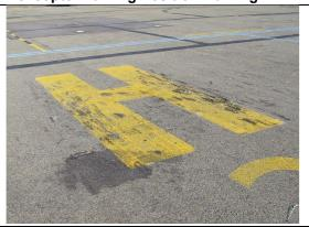
Helicopter parking position markings are areas specifically for helicopter parking. No other vehicle or aircraft is permitted to park in this area.
