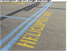
These lines define an area specifically for helicopter operations. These areas are defined by double solid blue lines and the text HELICOPTERS ONLY.
