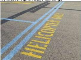
These lines define an area specifically for helicopter operations. These areas are defined by double solid blue lines and the text HELICOPTERS ONLY.
